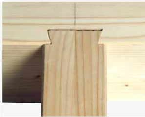
Dovetailed joints on floor joists or rafter (roof system)
